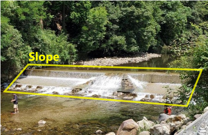
Fig. : Weir with a slope on the Muro River in Nara Prefecture
